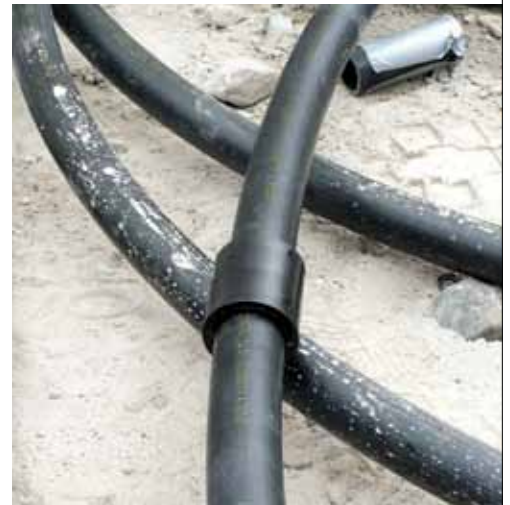
Typical thermally welded coupling for horizontal geo-exchange pipe.
